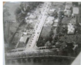
Figure 2.19: An aerial view of Colpin Ave and the Ideal Homes ? taken from a plane ?hired? for the purpose on 25/11/1933. - Ballarat Heritage Precincts Study, 2006
