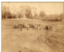
Chinamans Lagoon during construction 1878
