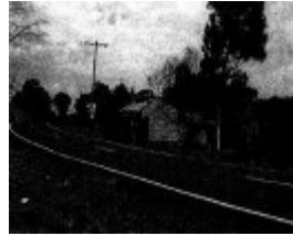
HO251- Jones farmhouse and outbuildings 2006
