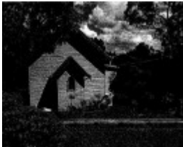
HO250 - Church - view from north (image from survey)
