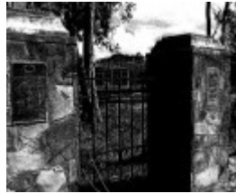
HO249 - detail of pedestrian gate
