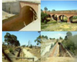
1 main outfall sewer collage
