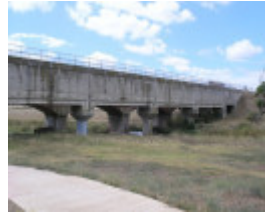
MAIN OUTFALL SEWER SOHE 2008
