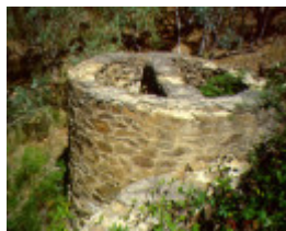
1 mt hepburn treatment works stone pier db
