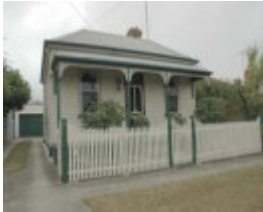
Photo No. 150305-143 - Ballarat Heritage Precincts Study, 2006
