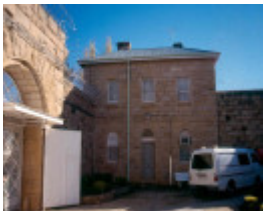
h01549 h m prison william street beechworth gaolers quarters and entry yard june2004
