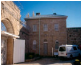
h01549 h m prison william street beechworth gaolers quarters and entry yard june2004
