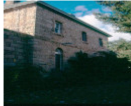
h01549 h m prison william street beechworth exterior gaolers quarters june2004
