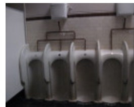
Warragul Railway Station urinals
