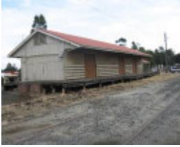
Warragul railway station goods shed from east
