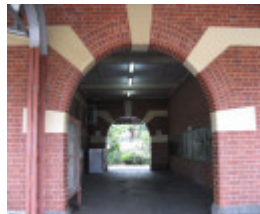
Warragul Railway Station link between 2 platforms
