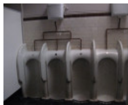
Warragul Railway Station urinals
