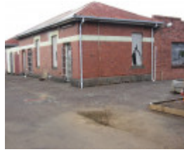
Warragul Railway Station drivers room
