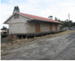
Warragul railway station goods shed from east
