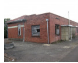
Warragul Railway Station drivers room addition
