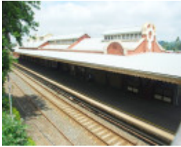
WARRAGUL RAILWAY STATION SOHE 2008
