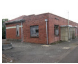
Warragul Railway Station drivers room addition
