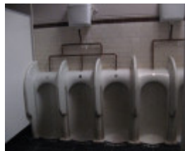
Warragul Railway Station urinals
