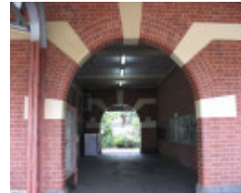
Warragul Railway Station link between 2 platforms
