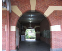
Warragul Railway Station link between 2 platforms
