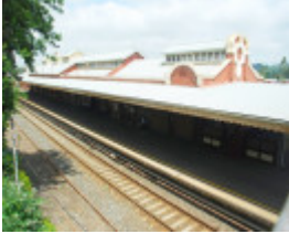
WARRAGUL RAILWAY STATION SOHE 2008
