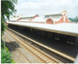
WARRAGUL RAILWAY STATION SOHE 2008
