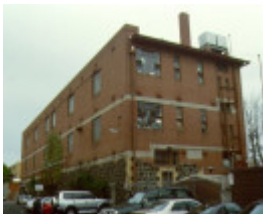
HER2001 001296 rvib st kilda rd factory workshop from north west 2001
