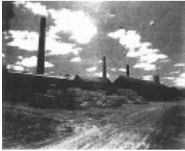
Darley Refractories Pty. Ltd.
