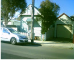
8 George Street, Geelong West
