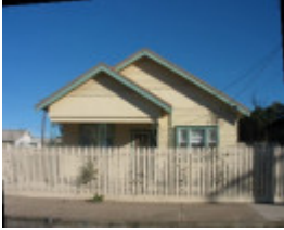
9 George Street, Geelong West
