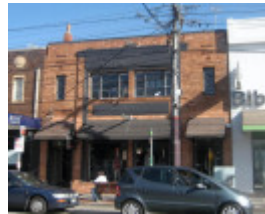
Former ES&A Bank, 510 Malvern Road
