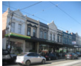
Victorian shops, 475-487 Malvern Road
