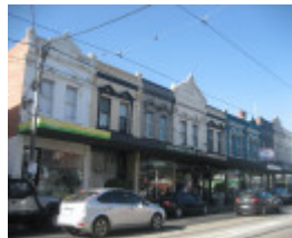
Victorian shops, 475-487 Malvern Road
