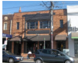
Former ES&A Bank, 510 Malvern Road
