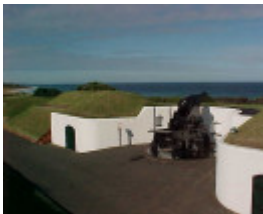
h01520 lady bay lighthouse complex battery jun04 pm1
