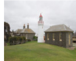
LADY BAY LIGHTHOUSE COMPLEX SOHE 2008
