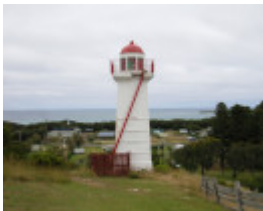
LADY BAY LIGHTHOUSE COMPLEX SOHE 2008
