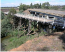
TRESTLE BRIDGE SOHE 2008
