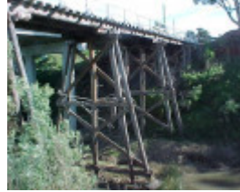
1 trestle bridge toward new bridge may01
