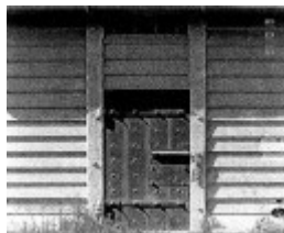
Portable timber lock-up. Main rd Eltham - Shire of Eltham Heritage Study, 1992
