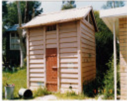
Portable timber lock-up. Main rd Eltham Colour 1 - Shire of Eltham Heritage Study, 1992
