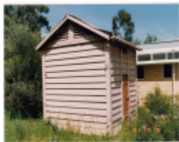
Portable timber lock-up. Main rd Eltham Colour 4 - Shire of Eltham Heritage Study, 1992
