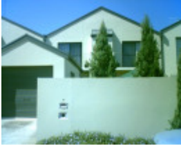
7 Potter Street, Geelong West
