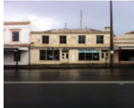
Appearance prior to repairs in 2013
