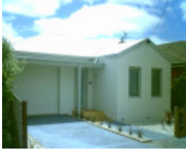
6-8 Pizer Street, Geelong West.jpg
