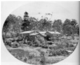
Southernwood rear view
