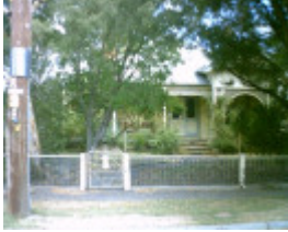
25-27 Lupton Street, Geelong West
