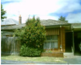
1 Plunkett Street, Geelong West
