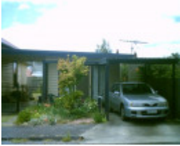
2 Plunkett Street, Geelong West
