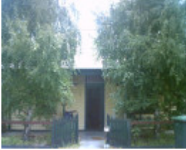
4 Plunkett Street, Geelong West
