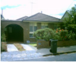
8 Plunkett Street, Geelong West
