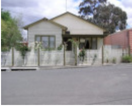
7 Arnott Street, Geelong West
