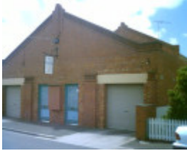
26-28 Potter Street, Geelong West
