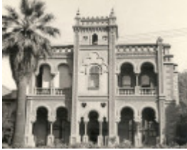
B0585 House East Melbourne
