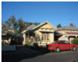
33a Wellington Street. Geelong West
