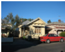
33a Wellington Street. Geelong West
