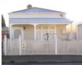
70 Preston Street, Geelong West
