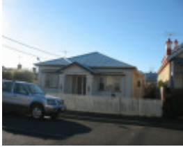
12 Tayler Street, Geelong West
