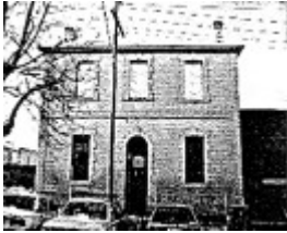
Gas Co Managers House - Ballarat Heritage Review, 1998
