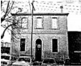
Gas Co Managers House - Ballarat Heritage Review, 1998
