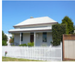
13 Flinders Street, Queenscliff
