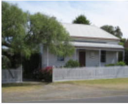
13 Flinders Street, Queenscliff
