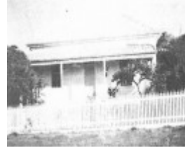
13 Flinders Street, Queenscliff
