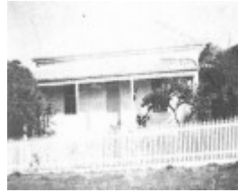
13 Flinders Street, Queenscliff
