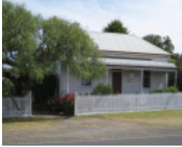
13 Flinders Street, Queenscliff
