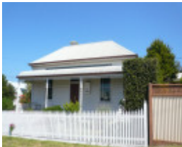
13 Flinders Street, Queenscliff
