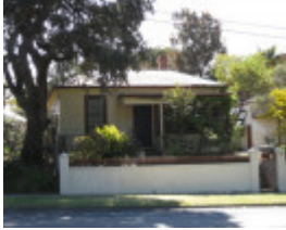
Neptune Cottage, 18 Gellibrand Street, Queenscliff
