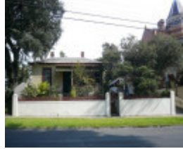
Neptune Cottage, 18 Gellibrand Street, Queenscliff
