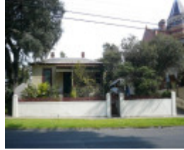
Neptune Cottage, 18 Gellibrand Street, Queenscliff
