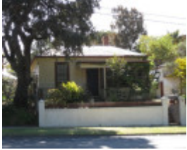
Neptune Cottage, 18 Gellibrand Street, Queenscliff
