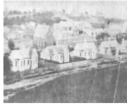
Health Officer's quarters on the corner of Stokes Street, and four of the original duplex cottages, c.1867 (Q.H.S. 14/251)
