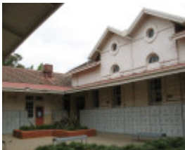
Bendigo Senior Secondary College_courtyard of 1914 building with remnants of 1870 building_KJ_Nov 09
