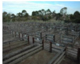
Overview of sheep pens showing introduced steel posts (former tram tracks) and horizontal timber rail.
