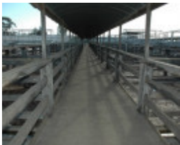
Details of covered way looking west.
