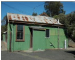
Market Offices building, north elevation
