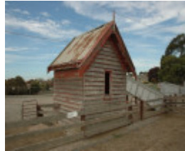
Former Caretaker's Cottage, west elevation
