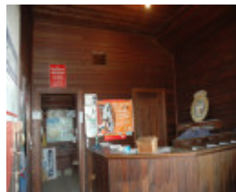
Interior HF Richardson office looking west. Note the early stained timber v-jointed ceiling and walls
