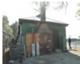
Market Offices building, south elevation
