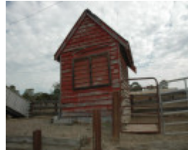
Former Caretaker's Cottage, east elevation
