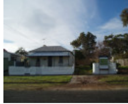
Stavely, 1 Henry Street, Queenscliff
