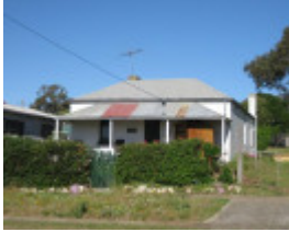
Stavely, 1 Henry Street, Queenscliff
