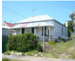
Stavely, 1 Henry Street, Queenscliff
