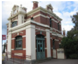
Queenscliff Post Office, 47 Hesse Street, Queenscliff
