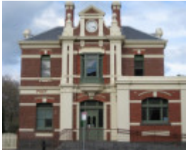
Queenscliff Post Office, 47 Hesse Street, Queenscliff
