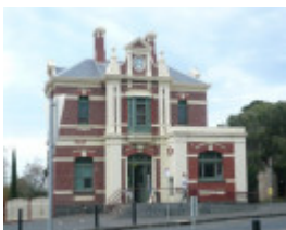
Queenscliff Post Office, 47 Hesse Street, Queenscliff
