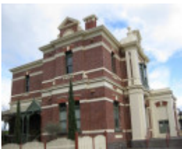
Queenscliff Post Office, 47 Hesse Street, Queenscliff
