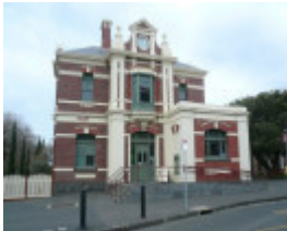
Queenscliff Post Office, 47 Hesse Street, Queenscliff
