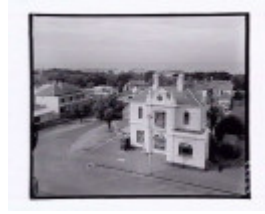
Queenscliff Post Office, 47 Hesse Street, Queenscliff
