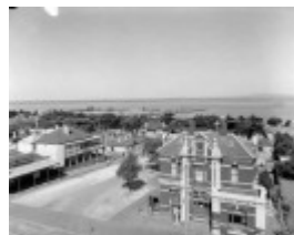
Queenscliff Post Office, 47 Hesse Street, Queenscliff
