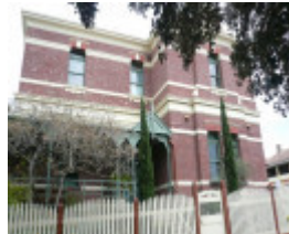
Queenscliff Post Office, 47 Hesse Street, Queenscliff
