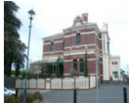
Queenscliff Post Office, 47 Hesse Street, Queenscliff
