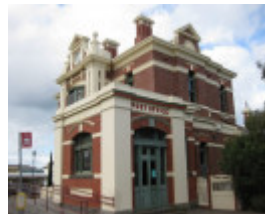
Queenscliff Post Office, 47 Hesse Street, Queenscliff
