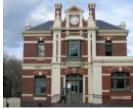
Queenscliff Post Office, 47 Hesse Street, Queenscliff
