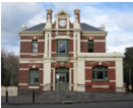
Queenscliff Post Office, 47 Hesse Street, Queenscliff
