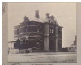
Queenscliff Post Office, 47 Hesse Street, Queenscliff
