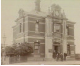
Queenscliff Post Office, 47 Hesse Street, Queenscliff
