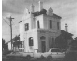
Queenscliff Post Office
