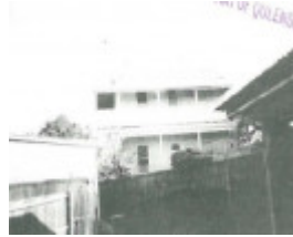
Oceania House, c.1888. (North facade)
