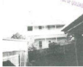
Oceania House, c.1888. (North facade)
