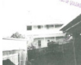
Oceania House, c.1888. (North facade)
