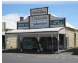
Former Bank of Victoria, 76 Hesse Street, Queenscliff
