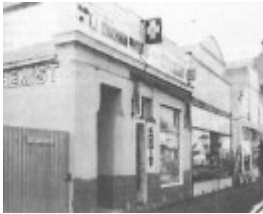
Former Bank of Victoria, 76 Hesse Street, Queenscliff
