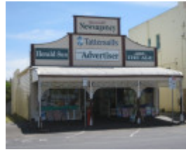
Former Bank of Victoria, 76 Hesse Street, Queenscliff
