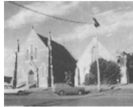
Former Wesleyan Churches, 79 -81 Hesse Street, Queenscliff
