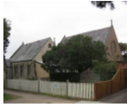
Former Wesleyan Churches, 79 -81 Hesse Street, Queenscliff
