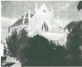
St Andrews Uniting Church, 83-89 Hesse Street
