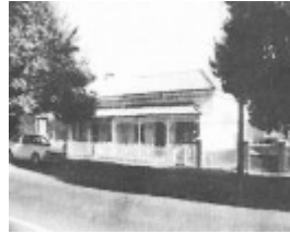
Warley and Shenfield Cottages.
