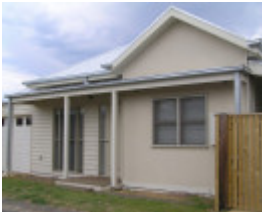
rear of 95 Hesse Street, Queenscliff
