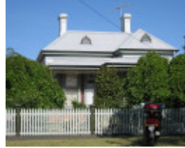
Carnbrea, 95 Hesse Street, Queenscliff
