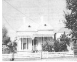
Carnbrea, 95 Hesse Street, Queenscliff
