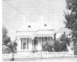
Carnbrea, 95 Hesse Street, Queenscliff
