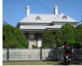
Carnbrea, 95 Hesse Street, Queenscliff
