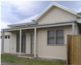
rear of 95 Hesse Street, Queenscliff
