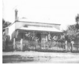
Navestock, 107 Hesse Street, Queenscliff
