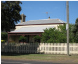
Navestock, 107 Hesse Street, Queenscliff
