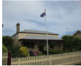
Navestock, 107 Hesse Street, Queenscliff
