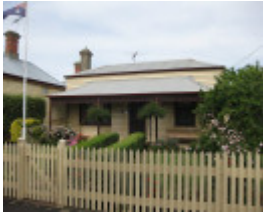
Navestock, 107 Hesse Street, Queenscliff
