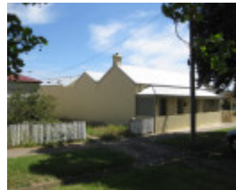
39 King Street, Queenscliff
