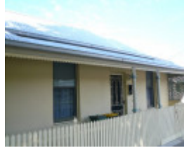
39 King Street, Queenscliff
