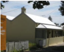
39 King Street, Queenscliff
