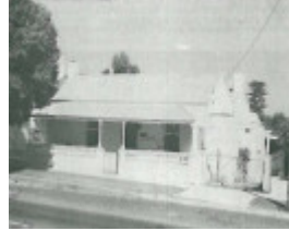
39 King Street, Queenscliff
