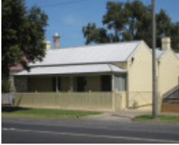
39 King Street, Queenscliff
