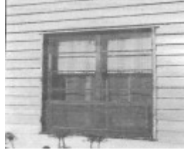
A ten-pane single sash window which disappears into the wall above when opened.
